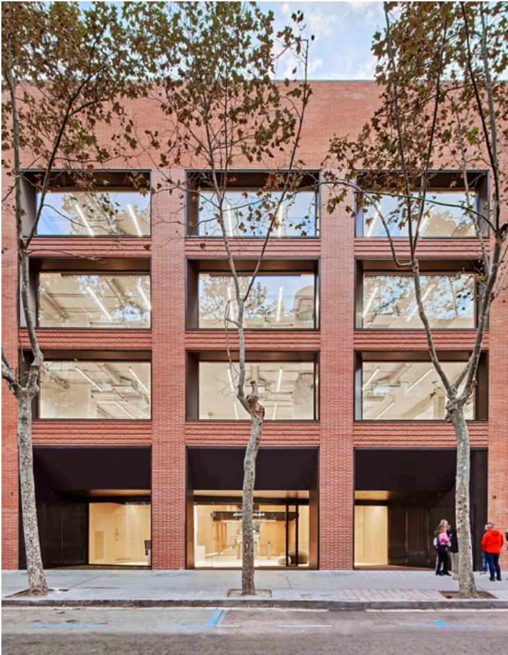
Commercial building, Joan Miro Spain
