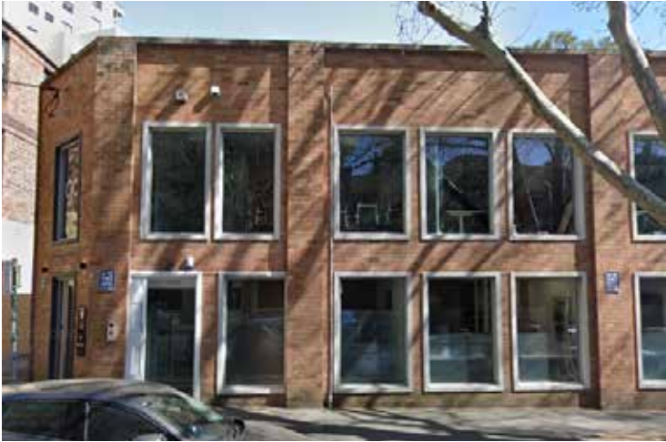
Brick facade of 33-39 Riley Street
