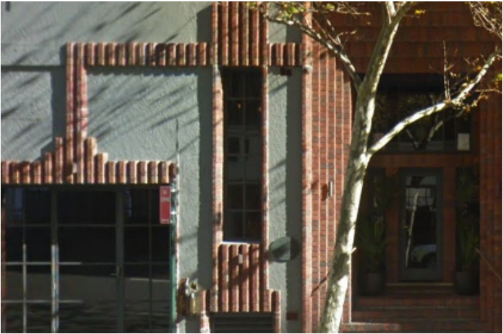
Brick detailing on facade of 55 Riley Street
